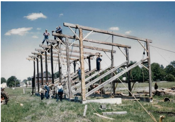
Rebuilding grandstand June 1957.
