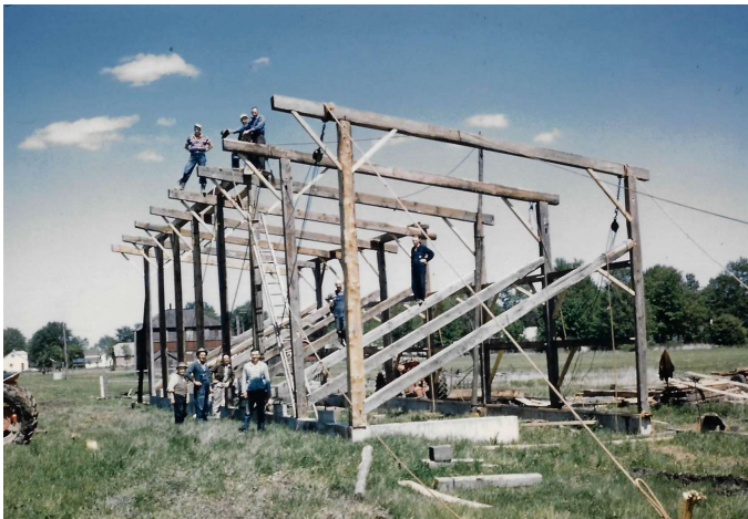
Rebuilding grandstand June 1957.
