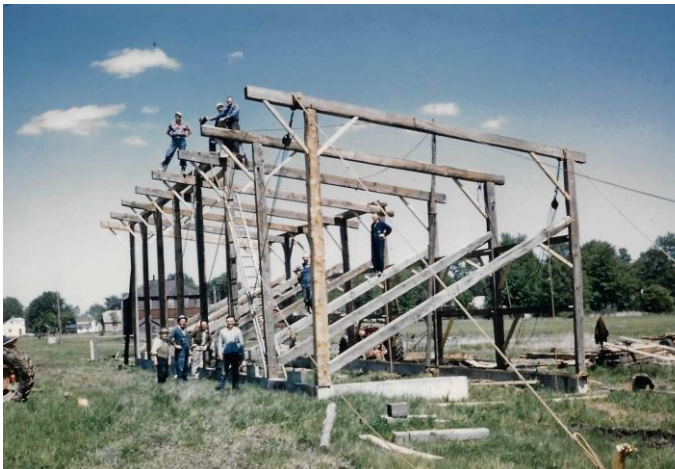
Rebuilding grandstand June 1957.
